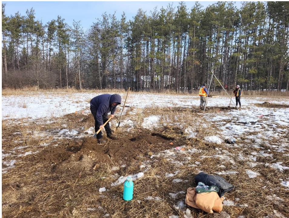
Image 2: Stage 3 excavations in progress; facing east, November 24, 2022.
